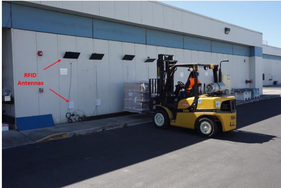
Figure 18: Meter Storage Area
