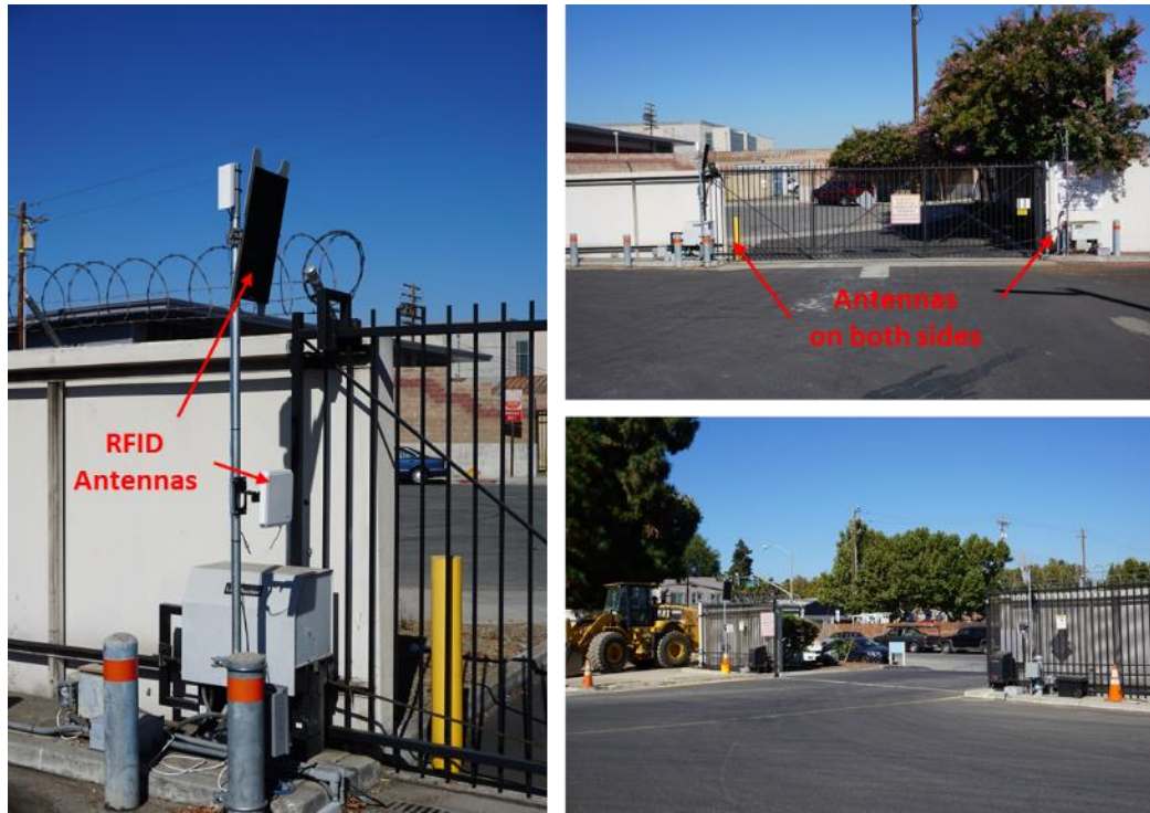
Figure 17: RFID Readers on Yard Gates
