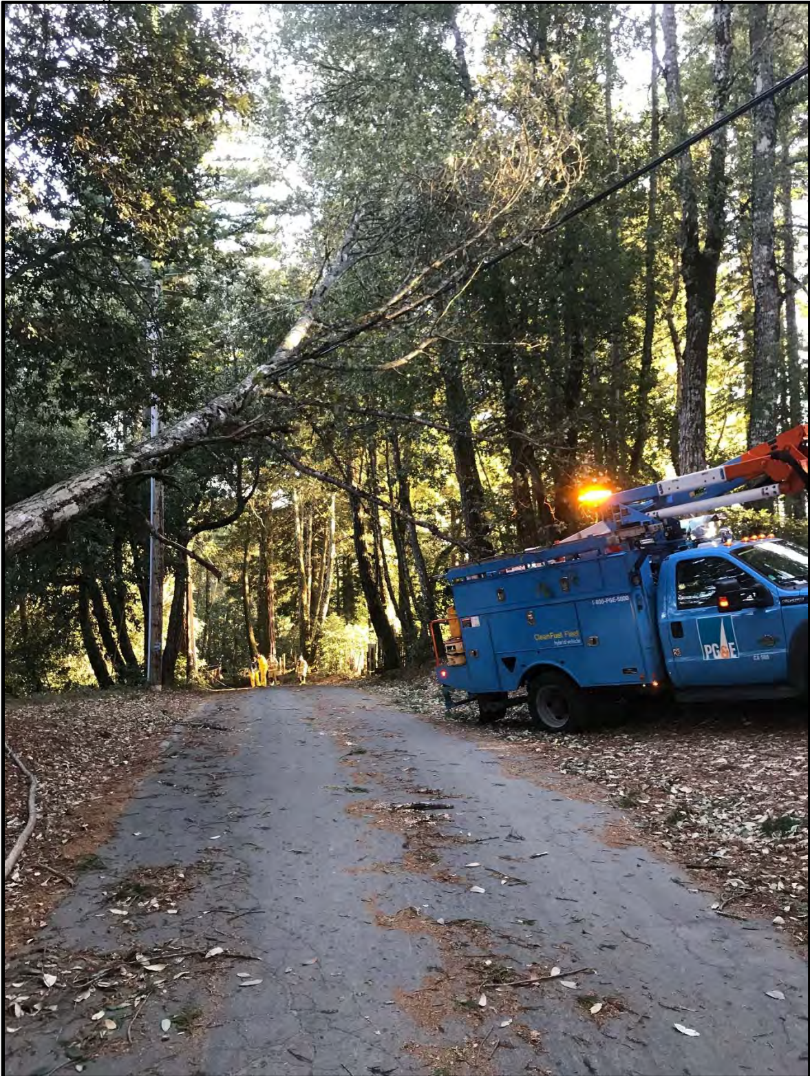
Figure 3: Tree fell onto conductors; Watsonville, Santa Cruz County
