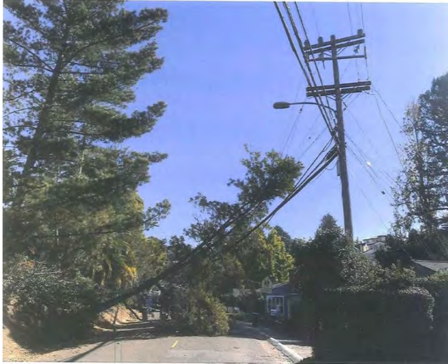
Figure 4: Tree fell on to conductors in Oakland, Alameda County
