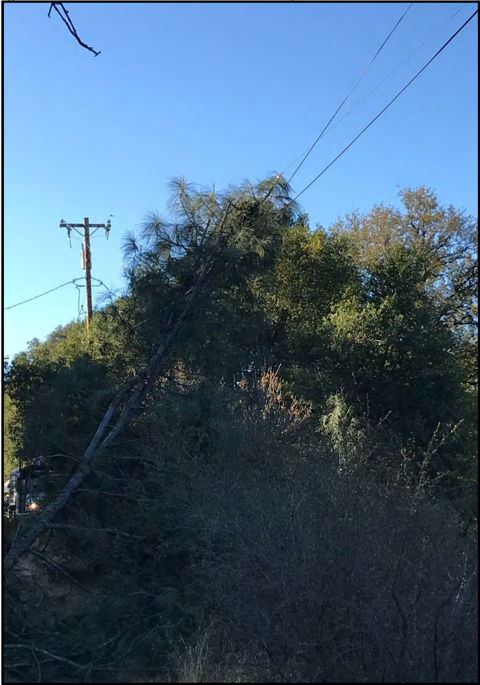
Figure 5: Tree fell onto conductors; Unincorporated area of Lake County
